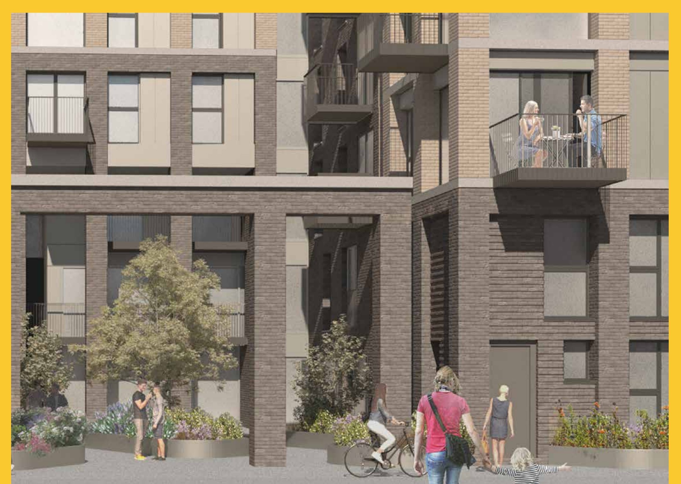
▶ BROWN TONED BRICK TO BASE ELEMENTS, GRID FORMED WITH BUFF TONED BRICKWORK, PRECAST STRING COURSES AND ALUMINIUM INSET PANELS
